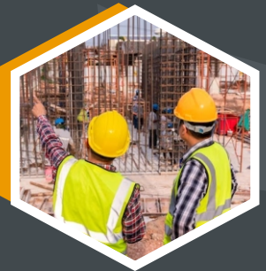
Civil Construction works
