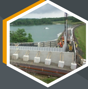
Civil works in fly ash pond
